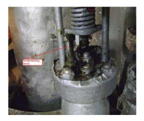
QCV blocked utilizing a bolt to hold in the open position. (Note: the painted portion on the bolt indicating possible long term condition.)
