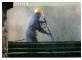
Fig. 5 High-pressure water washing of an actual block.
