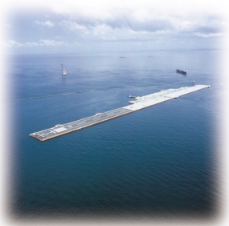
MEGA-FLOAT test model structure (1000m × 120m [max.] × 3m)
