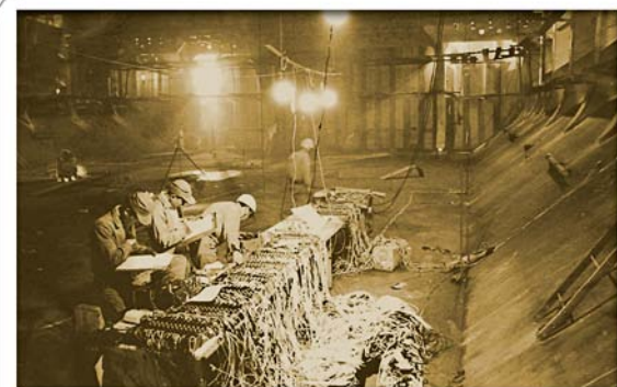
Full-scale measurement for double-bottom construction of a cargo ship in 1964.
