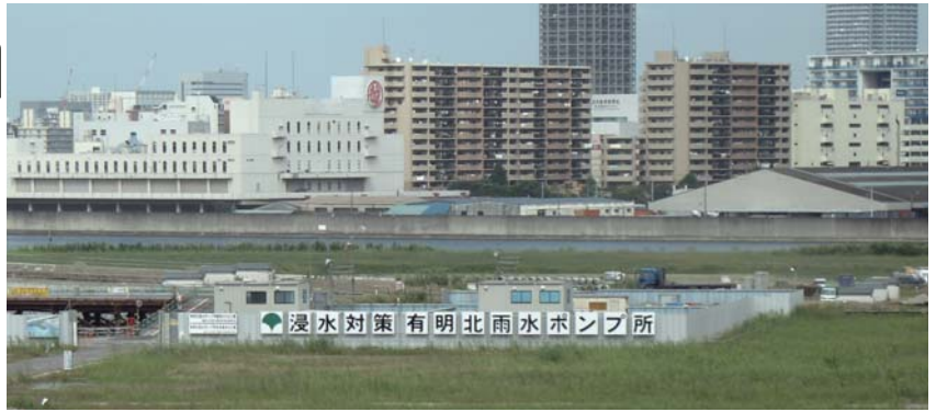
Water pumping station on reclaimed land in Tokyo bay
