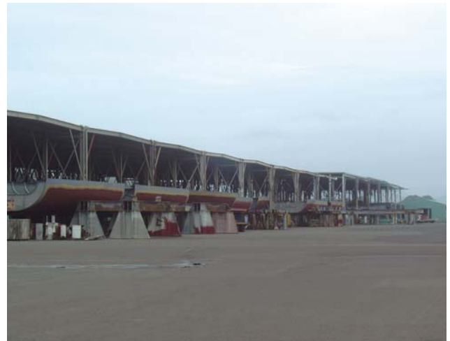
Hull block production at Oshima Shipyard
