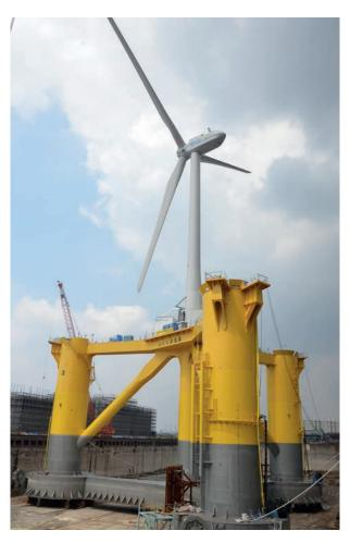
Fukushima future: 2MW offshore floating wind turbine generation facility
